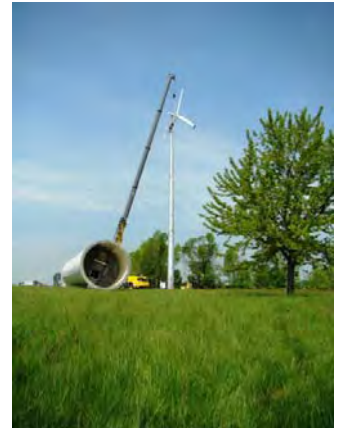
Rescue Tower & Entegrity Turbine
